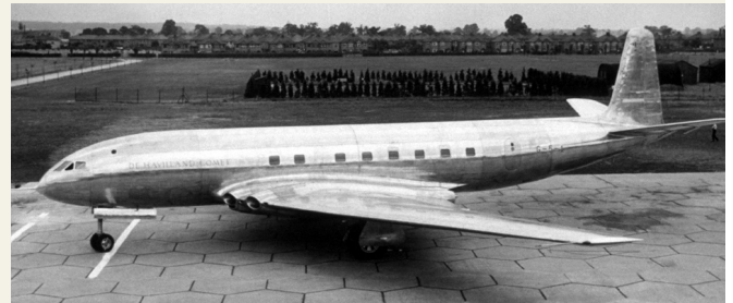
Figure 9. The de Havilland Company of England designed the first commercial jet airliner, the Comet. It first flew in 1949 and entered service in 1952. The Boeing 707 prototype did not fly until 1954. Credit: Getty.
